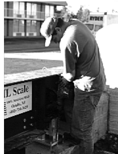
Figure 5-2. Install Anchor Bolts
