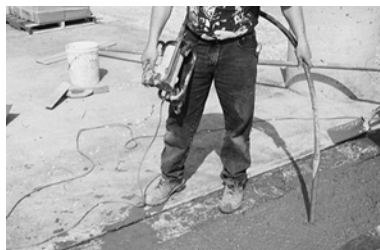
Figure 7-3. Concrete Vibrator
