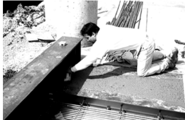
Figure 7-5. Finish Against Siderails
